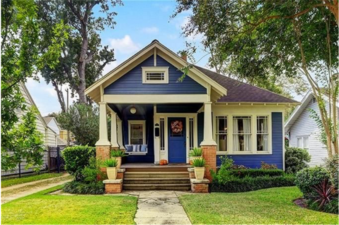
A smaller arts and crafts cottage with a prominent porch and entranceway, brick column bases, wooden columns, beams and knee braces with broad wood trim boards at top of walls
