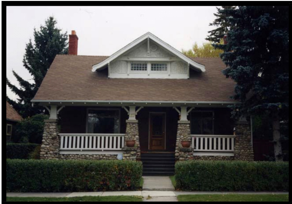
An original Craftsman – note the columns, the flat 2x8 railing pickets, stonework, gabled second floor window, knee braces, large and deep porch, steep roof slope.
