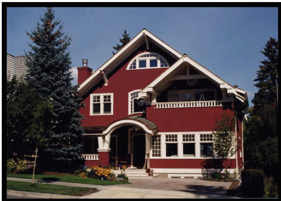
Note the entry porch, roof, double columns on a broad stucco base; wide door & window casings; knee braces, grouped windows, repetition of window style with small paned mullions; curved window treatment, beams & columns supporting the deep roof overhangs
