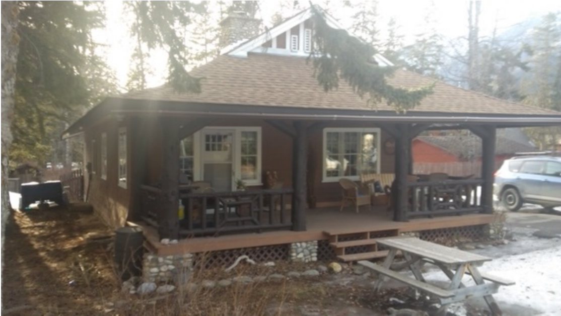
A rustic timber frame cottage in Banff – columns, beams, angle braces, heavier timber railing with a decorative center portion, deep porch and steep roof with a dormer at the top
