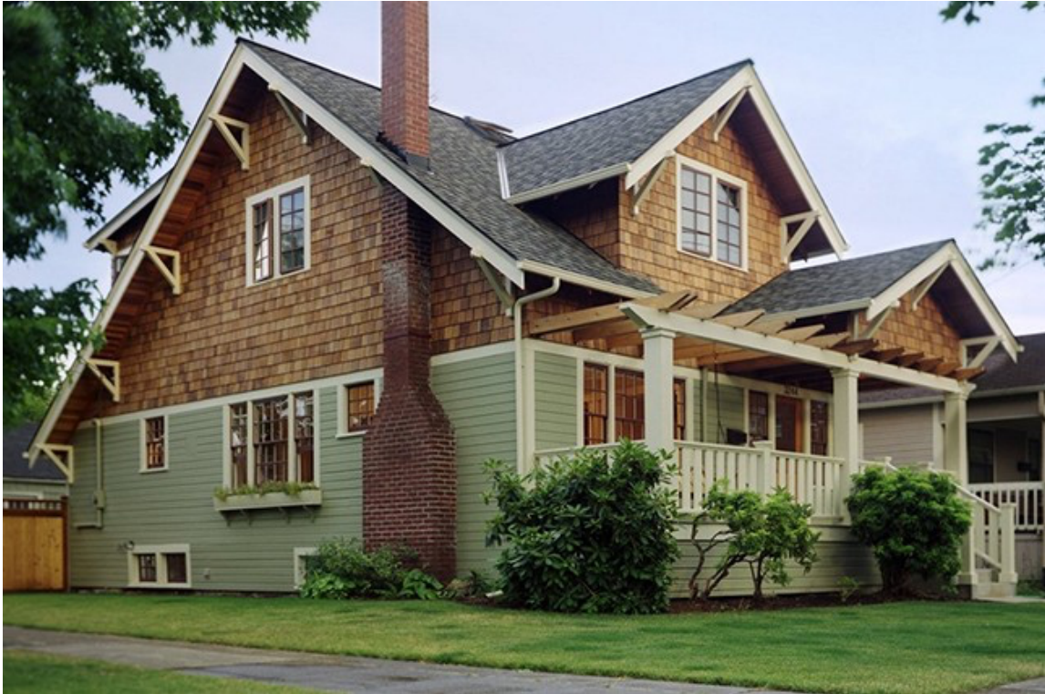
This is luxurious newer home in the arts and crafts style with wide porch, grand entry, shingles accenting the second floor, knee braces, columns and beams with steeply pitched roof
