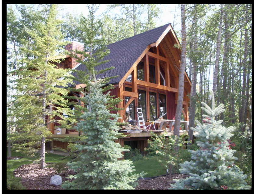
This cottage can be seen at Meridian Beach by the main boat launch and is a fine example of timber frame construction
